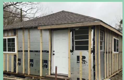
External Insulation
