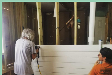
Shiplap - "No Drywall House"
